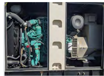
EASY ACCESS FOR MAINTENANCE
